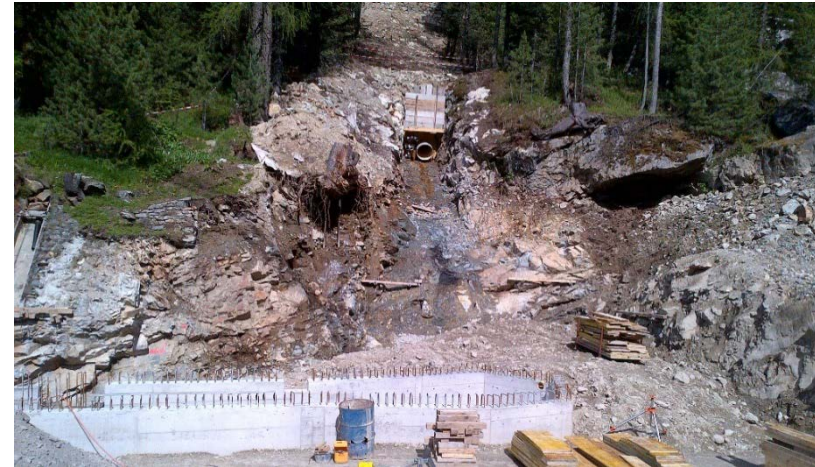
Construction at Morteratsch plant: pressure line (back) and underwater canal/powerhouse (front)
