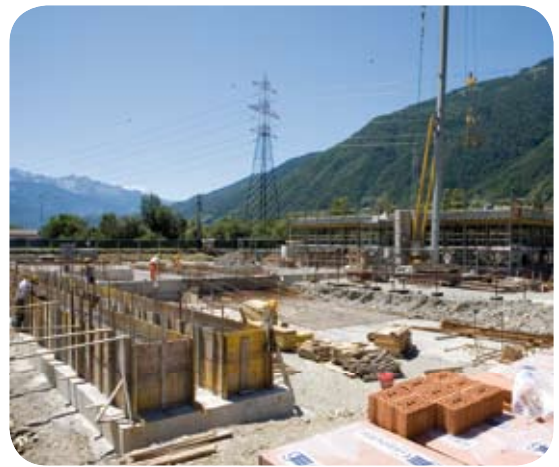
Investments in cross-border energy exchange: construction has begun in Tirano.
