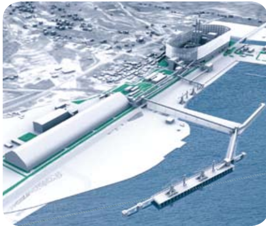
An architectural simulation of the Saline Joniche power plant: a pier for coal ships can be seen in the foreground with the covered coal storage facility to the left and the actual power plant on the right.
