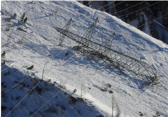
Job from Swissgrid: high-voltage pylon destroyed by avalanche on the Fuorn Pass, Zernez
